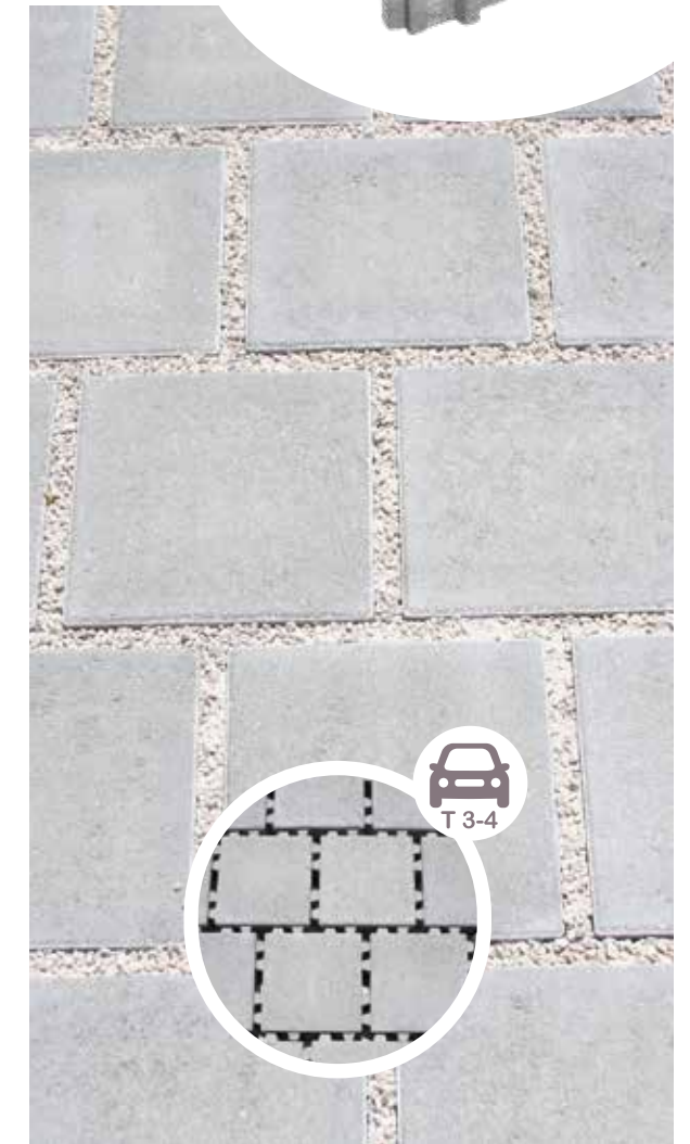
Pose joints croisés = CIRCULABLE T3-4
